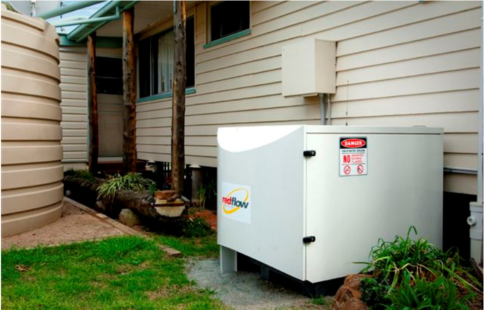
The Power+BOS® energy storage system is packaged in a utility-grade steel enclosure with a non-rusting base. Close inspection of this photo shows the 3G antenna mounted on the enclosure. This is used for data communications back to RedFlow's facility in Brisbane.
